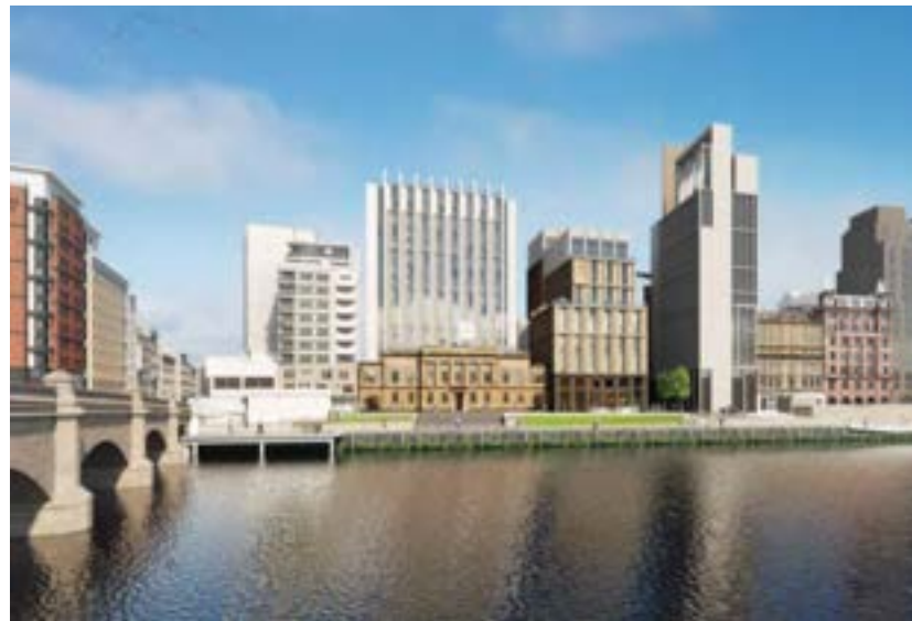
Custom House - June 2018
