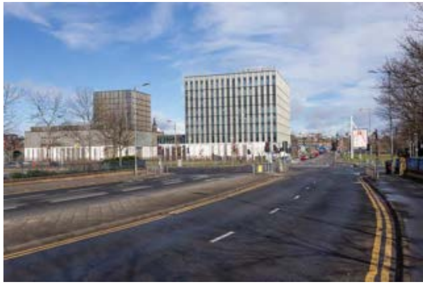
6 View from Crown Street across the river - looking North
