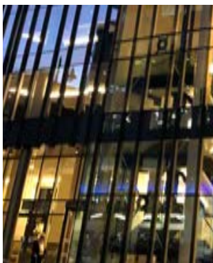
Glazing to lower and ground floors encourage active street frontage
