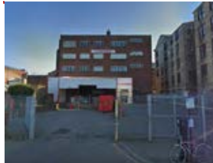
View to neighbouring warehouse building
