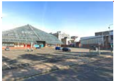
View towards St Enoch Shopping Centre
