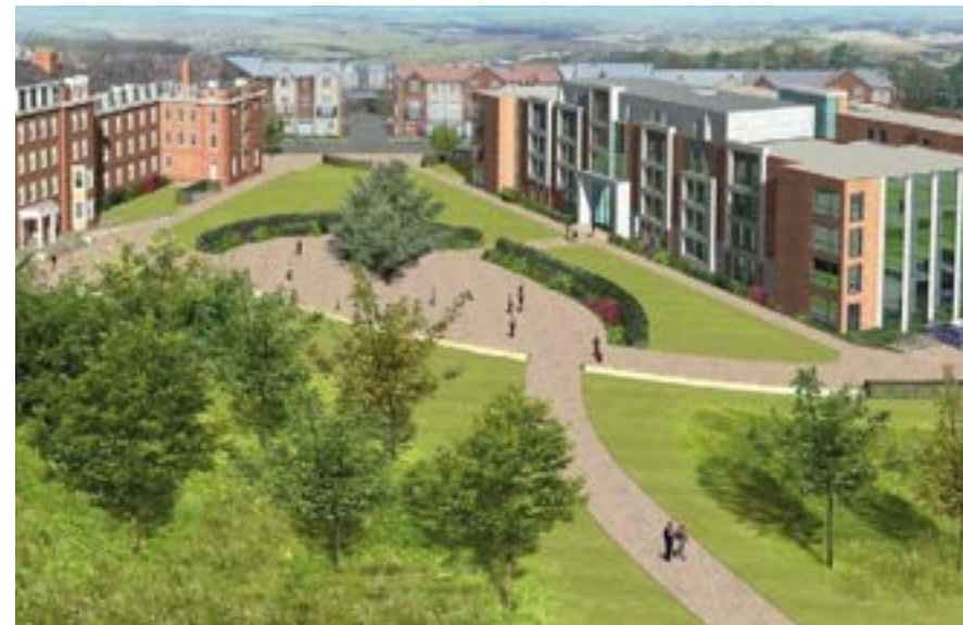
Sheraton Park, Durham (Howarth Litchfield Designed)
