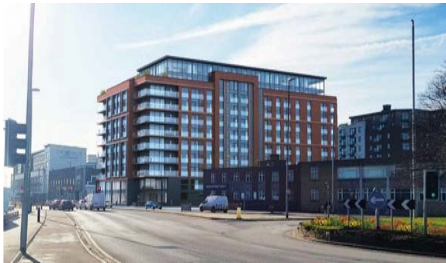
9 View from North Approach on A61
