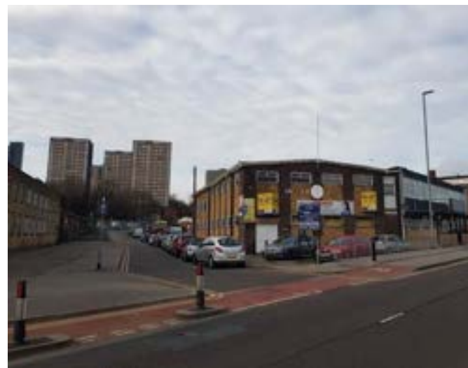
1 East Approach via Sheepscar Street South
