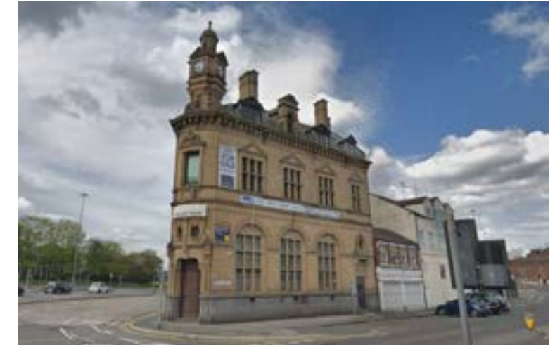
Northwood House, Grade II
