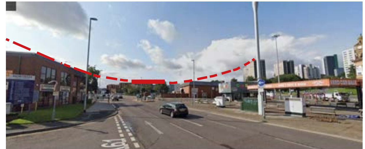
4 Long range view south along A61
