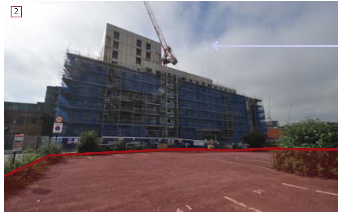
THE IRONWORKS (UNDER CONSTRUCTION) OPPOSITE SITE ON SCOTLAND STREET
