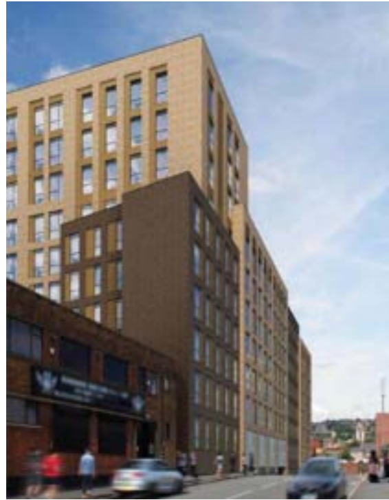
The Ironworks development Opposite site Apartments 6-10 storeys
