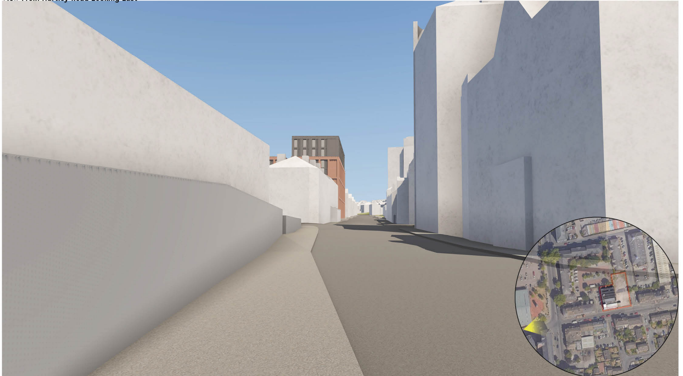
View From Hartley Road Looking East
