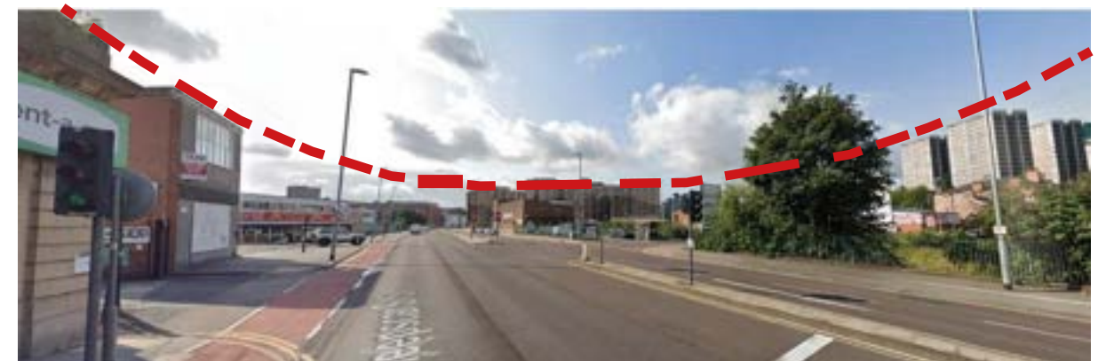
5 Mid range view south along A61
